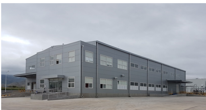
Solvay Performance Polyamides' new Technyl® compounding facility located in San Luis Potosí, a leading area for automobile production. Photo: Solvay Performance Polyamides
