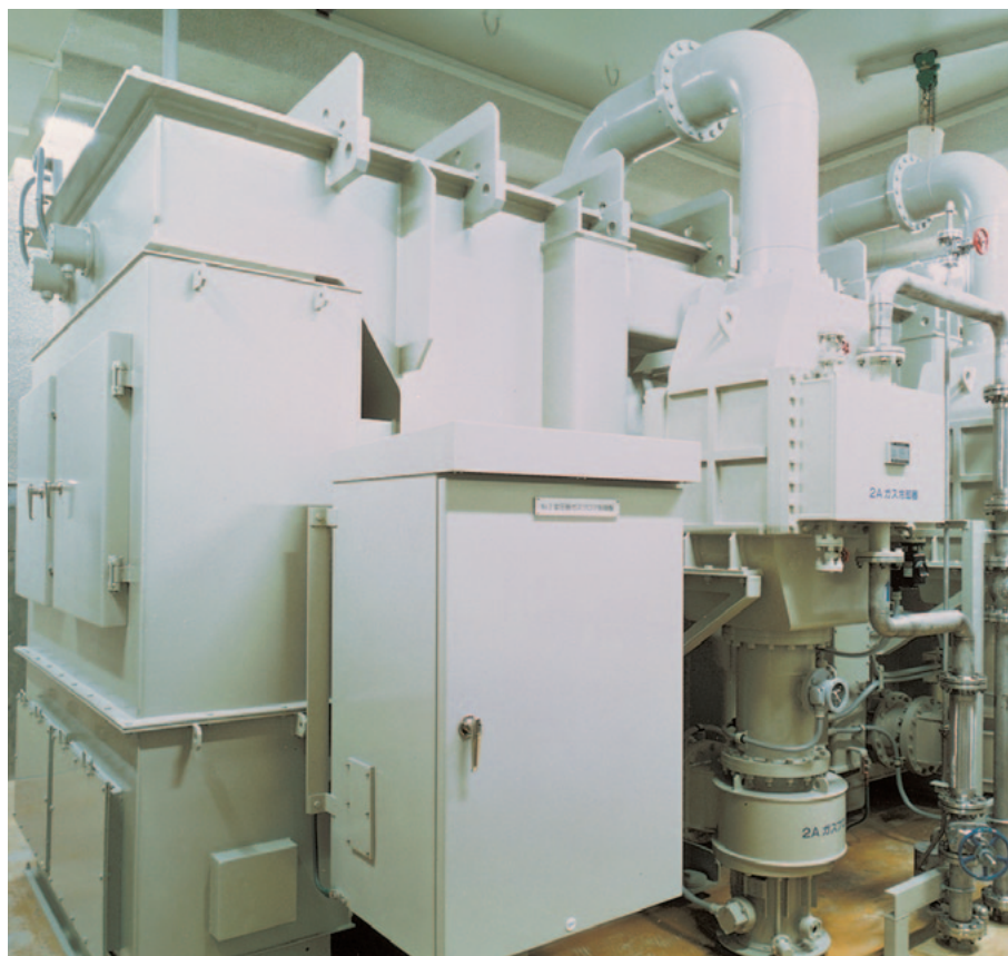
Fig. 17 \text{SF}_6 -insulated transformer, 23 – 107 kV (Fuji, Japan)
