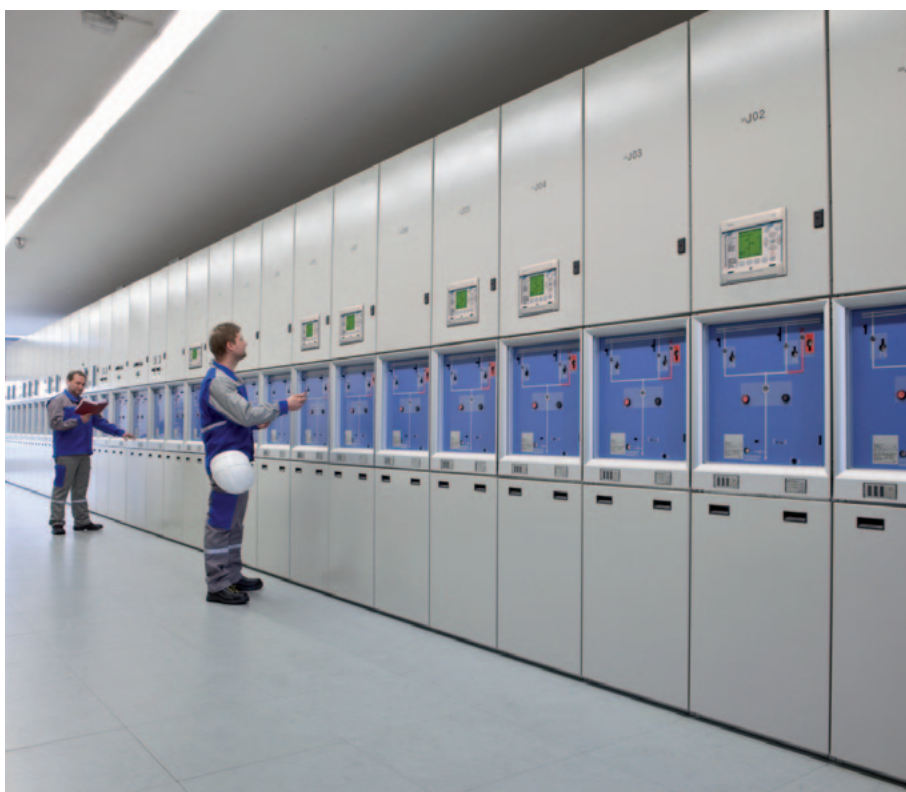
Fig. 13 Compact SF 6 -gas-insulated medium voltage switchgear, 40.5 kV as double busbar system (Schneider Electric, Germany)
