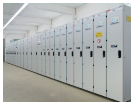
Fig. 14 SF 6 -gas-insulated medium voltage switchgear, 24 kV as double busbar system (ABB, Germany)
