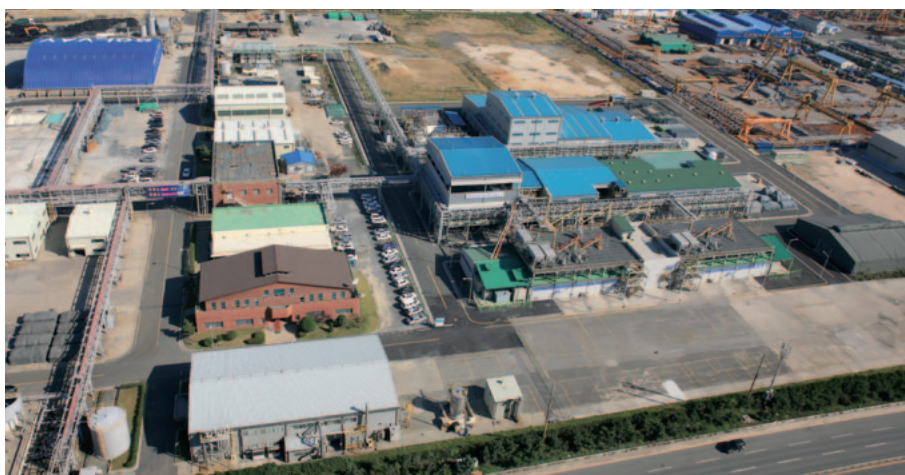
Fig. 59 Plant Onsan, South Korea
