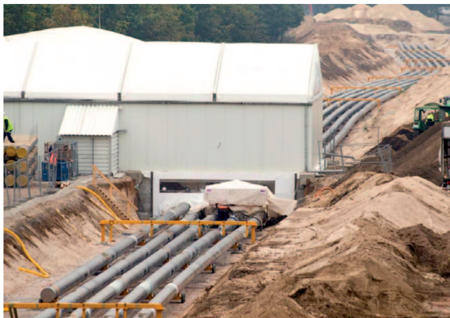
Fig. 10 Polyethylene coated GIL system for direct burial 245 – 550 kV (Siemens, Germany)
