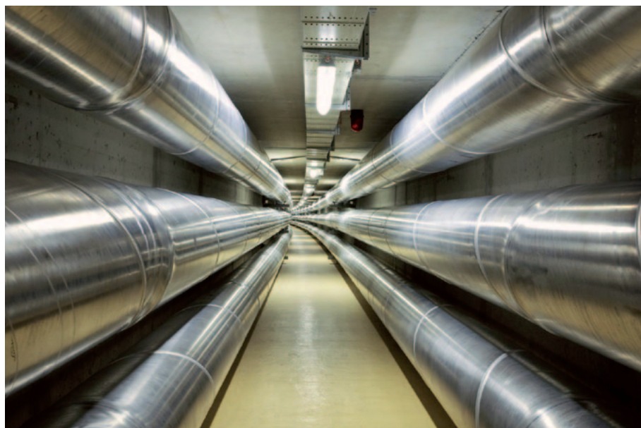
Fig. 11 Gas insulated line for \text{SF}_6/\text{N}_2 mixture in a tunnel 245 – 550 kV (Siemens, Germany)
