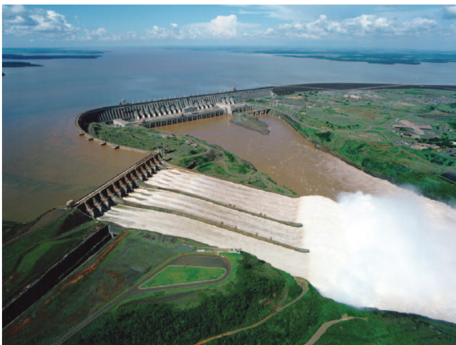
Fig. 8a Hydroelectric power station Itaipú, Brazil
