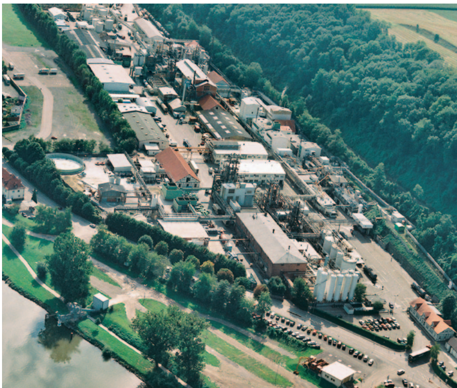
Fig. 58 Plant Bad Wimpfen, Germany
