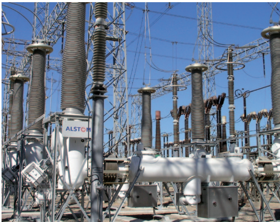
Fig. 4 SF 6 -insulated hybrid module, 420 kV (Alstom Grid, France)
