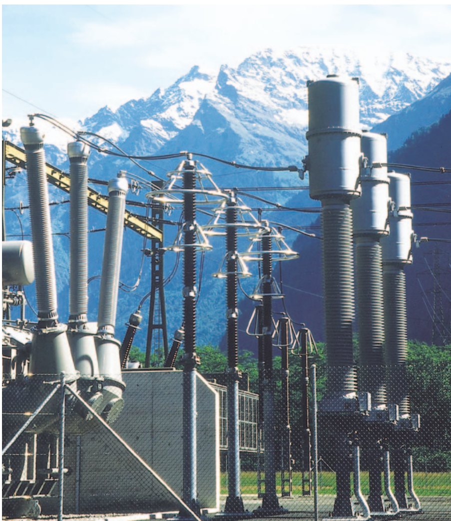
Fig. 18 \text{SF}_6 instrument-transformer, 420 kV (Trench Germany)
