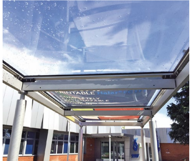
Halar® High Clarity ECTFE is being used for a covered walkway at Solvay Specialty Polymers' headquarters in Bollate, Italy.
