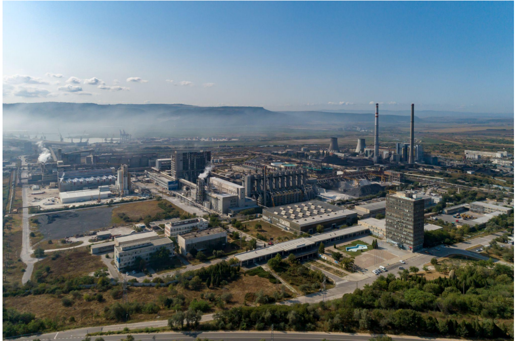
De fabriek van Solvay in Devnya © Solvay
