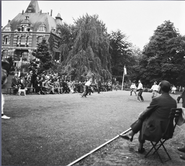
_Solvay Sport Balle Pelote field, Brussels, Belgium
