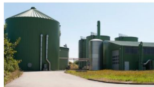
Biogas from agriculture 3 plants in France
